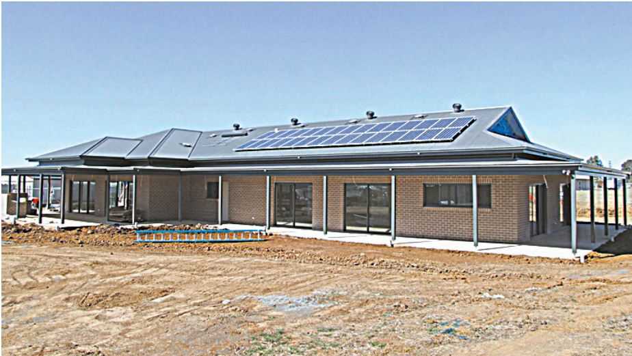
New home 5kw solar grid-connect installation
